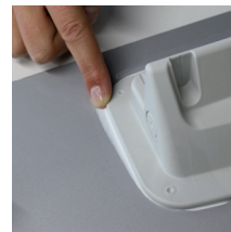
Step 11 Spray cleaner on your finger and spread it along the joints to even the joints.
