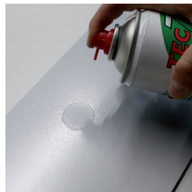
Step 7 Use cleaner for under-ground cleansing, no primer necessary.
